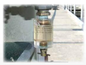
Des-Case® Desiccant Bladder Breathers were installed on the gearboxes to seal the gearbox from outside humidity and contamination.
